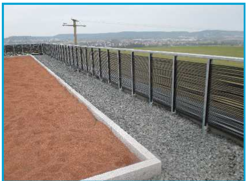
Absorber fencing designed as a rail system incorporating a privacy protection screen, e.g. for regeneration of ice storage systems or other applications (with special PE-pipes)
